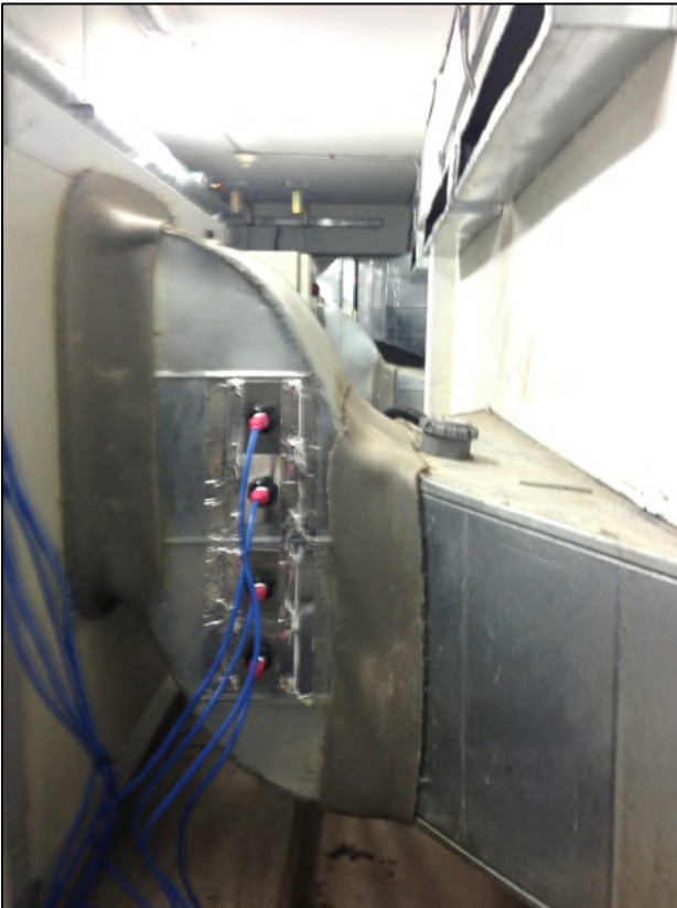
Left side of theatre 4 UV tube installation
