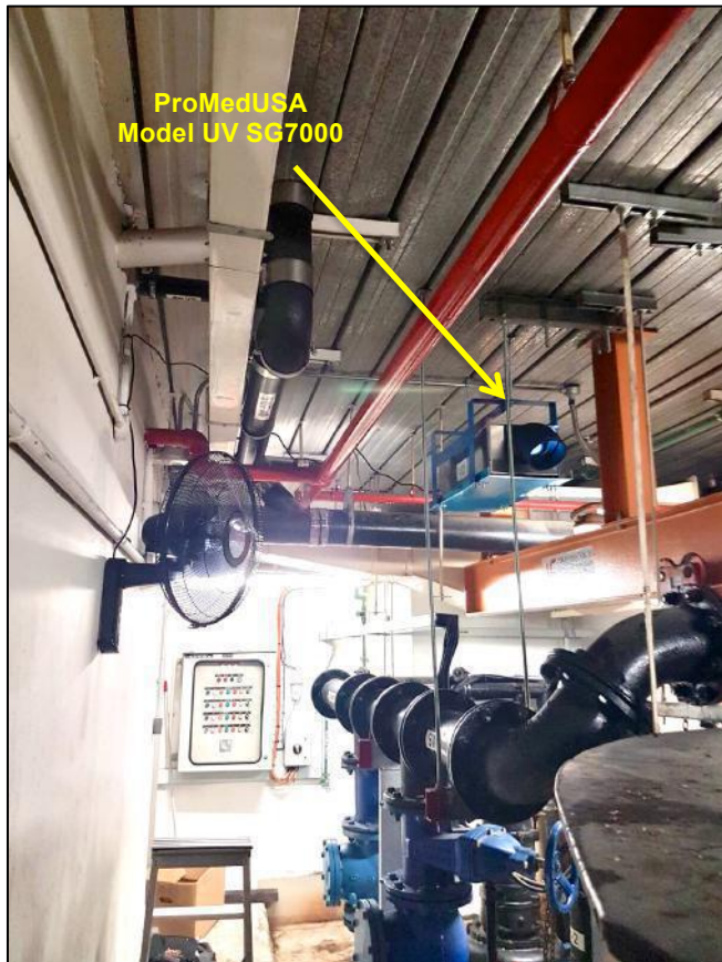
B2 level Grease Trap Room with one UV SG7000
